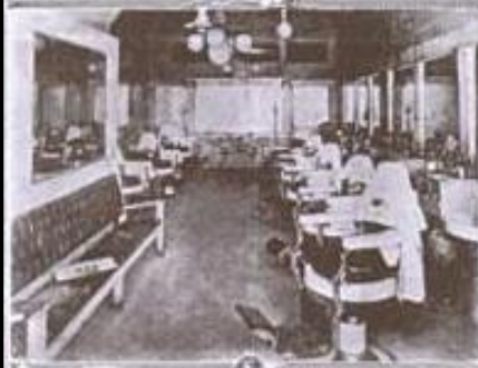
Master View of Shop at 7 North Broad Street
